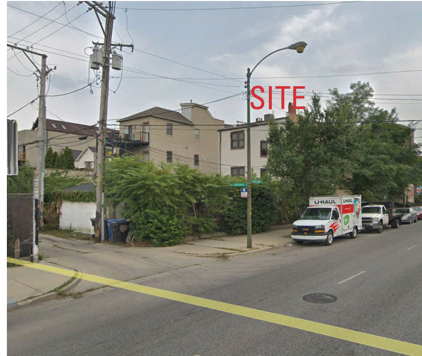
CORNER VIEW OF SITE LOOKING SOUTHEAST
