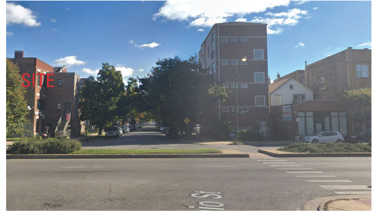
LOOKING EAST TOWARDS OHIO AT ASHLAND AVE AND SITE (RIGHT)
